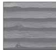
R. Wood Siding
